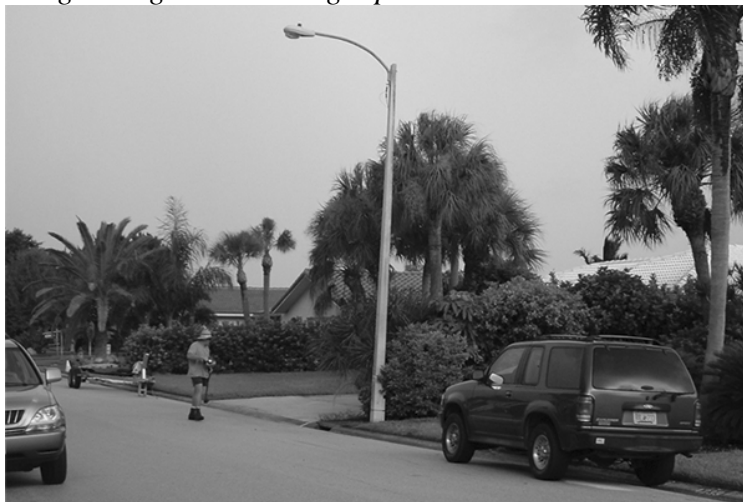
Newer style of “cobra-head” light pole. Note that pole is leaning
